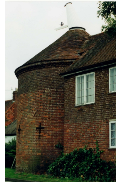
Circular red brick oast conversion with peg-tile roof
