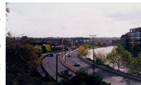
The A29 has carved a route through the northern part of the town
