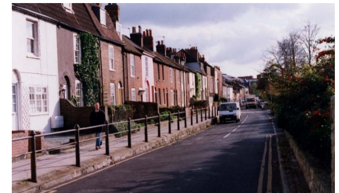
19th century terraced housing in north Maidstone
