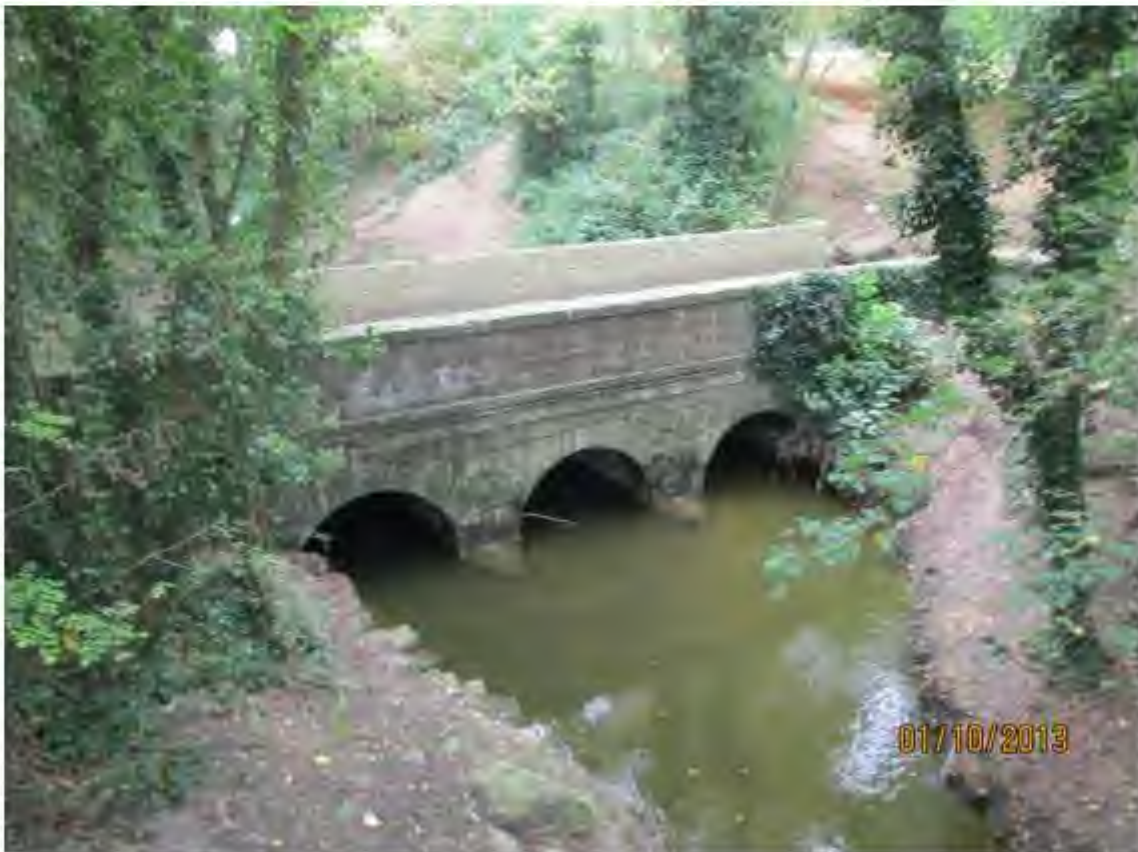
Photograph 13: West Ride bridge over existing spillway channel (control on flows)
