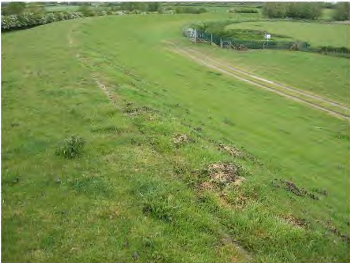
Photograph 2: Grass reinforced mat
