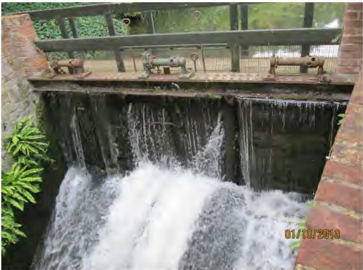
Photograph 19: Gates at end of Mill Race
