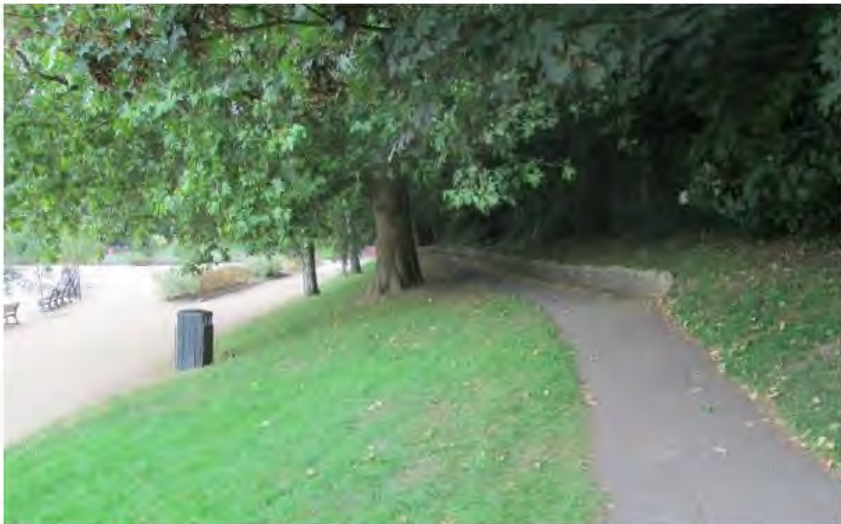
Photograph 9: East end of high level path; showing end of crest wall
