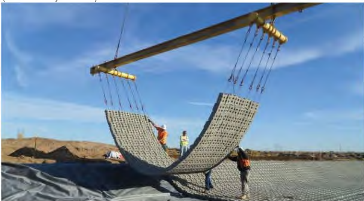
Photograph 4: Cable tied concrete block system (Armourflex by Contech)
