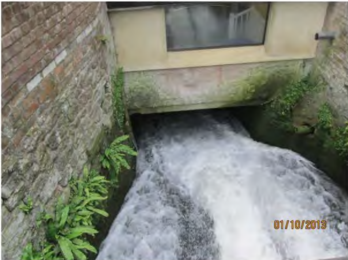
Photograph 21: View indicating floor level of Mill building well below level of Mill race
