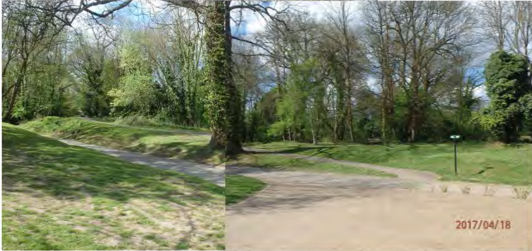
Photograph 14 View from upstream of position of Option C (holly covered stump on right is end is where fence runs up downstream face)
