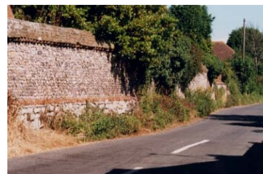
Red brick used to divide different materials
