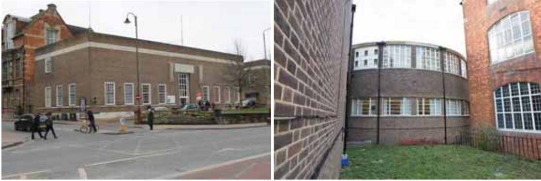
The main elevation and the bowed east elevation of the main library rooms
