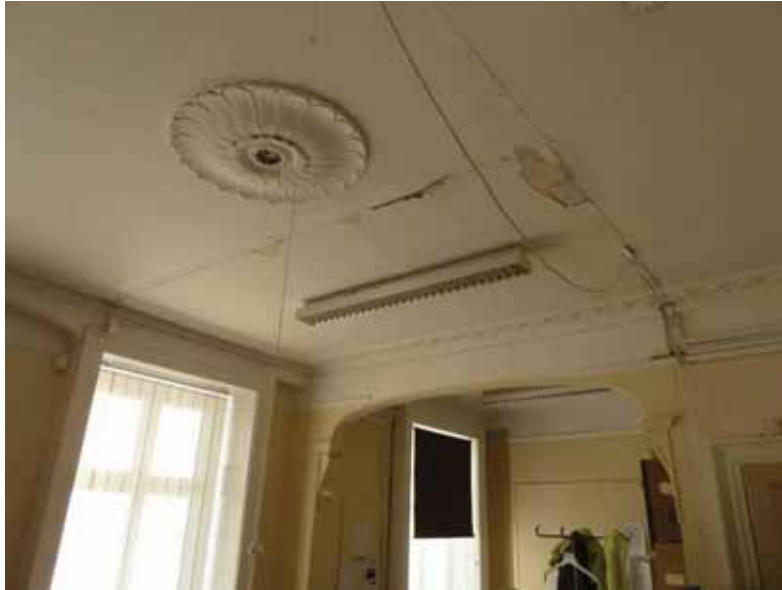
Ground-floor front room of no. 9
