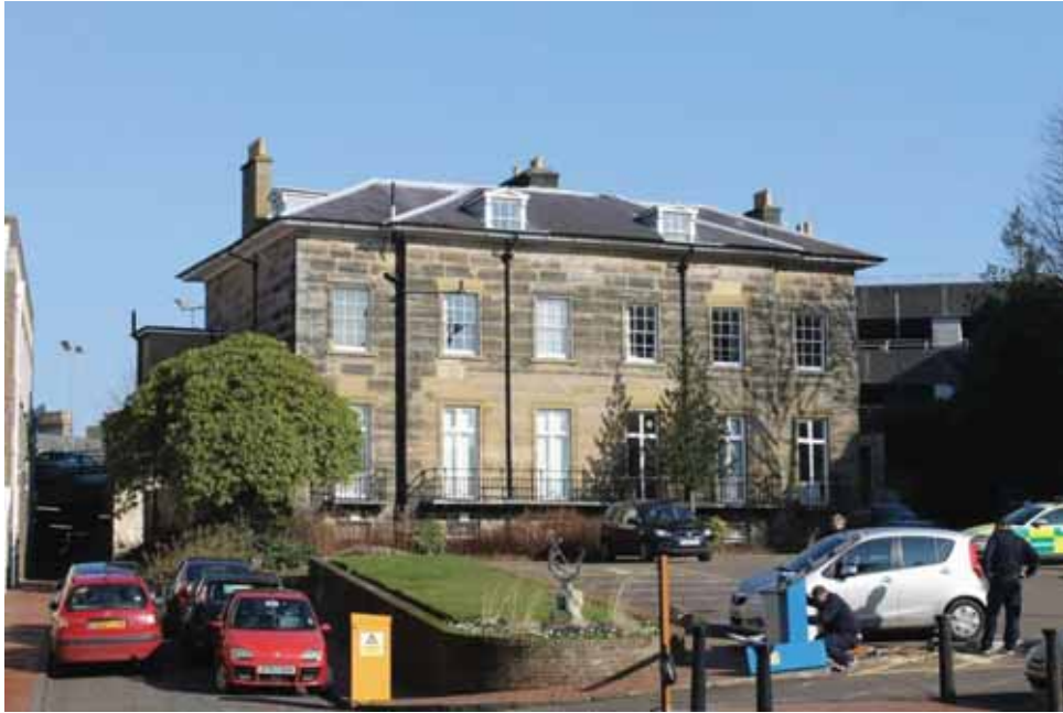
Exterior, from the southwest
