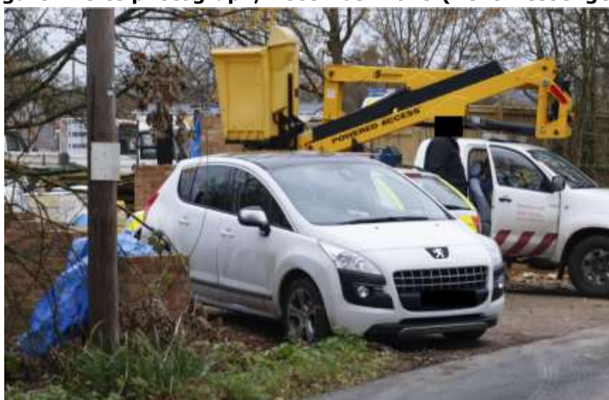
Figure 2: Site photograph, December 2015 (Kent Messenger).
