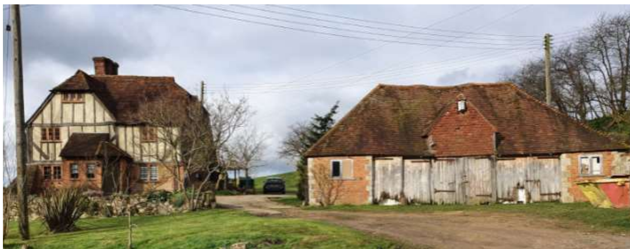
Figure 1: Photo of the barn and grade II listed Rosehill
