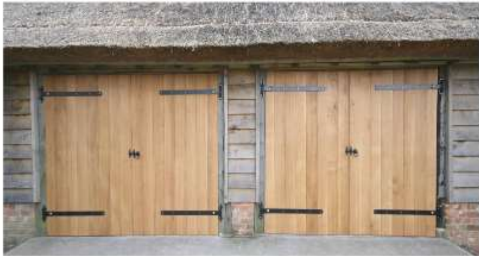
⑦ oak barn shutters/doors with cast steel hinges
