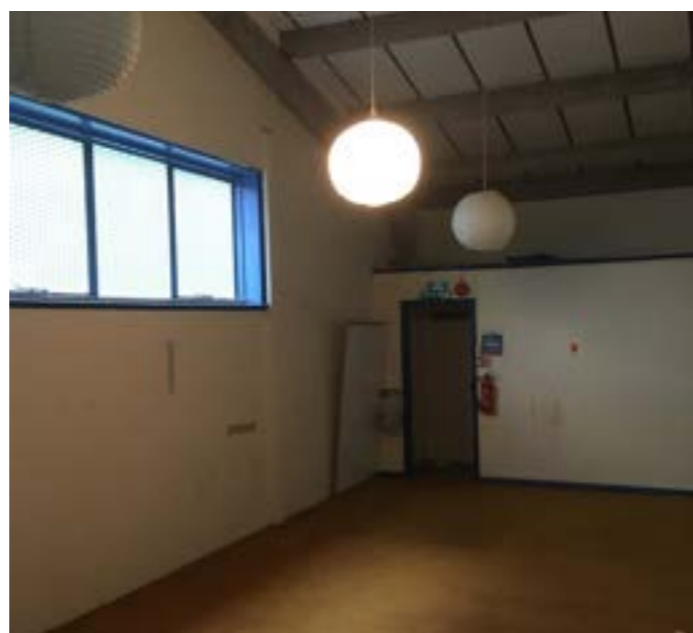
Image J- Unused first floor storage area
