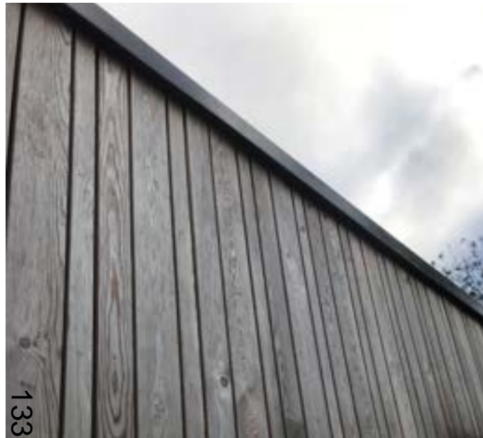
133 Heather House Site- Timber Cladding
