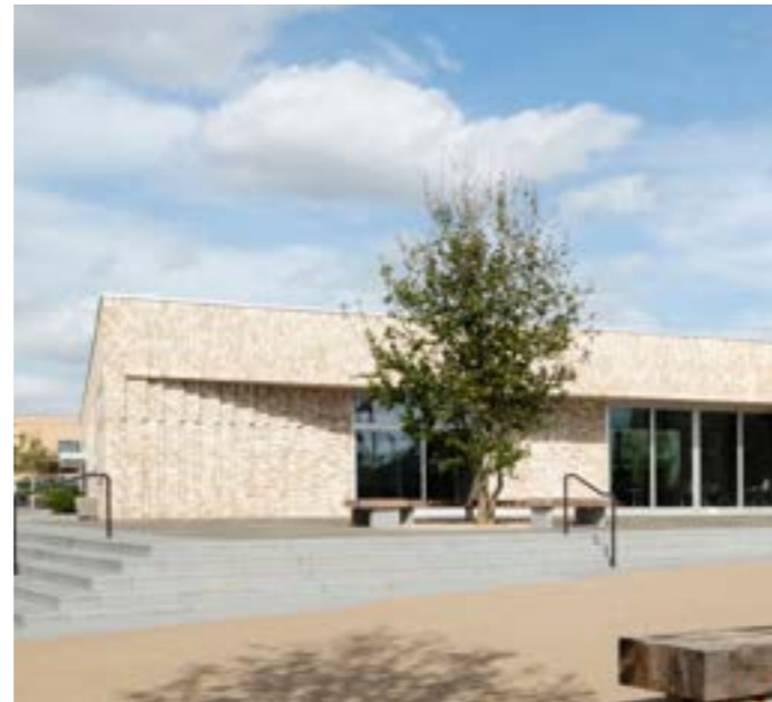
Heather House Site- Projecting Parapet
