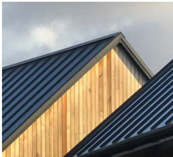
Pavilion Site- Standing Seam Roof
