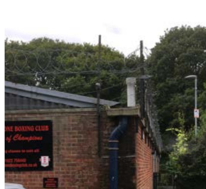
Image K- Security measures to prevent access to roof
