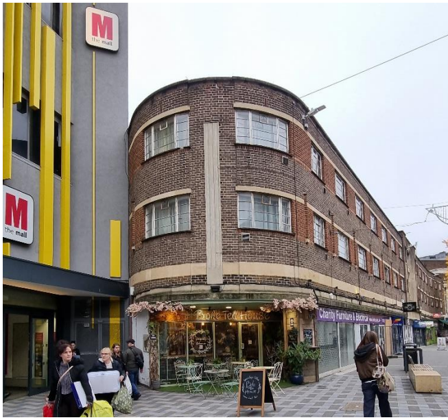
Figure 7 – Art Deco inspired building, with the Crittal windows above would suit metal shop front.
