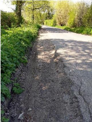
Damage from traffic to verge on Five Oak Lane close to Winery, causing ditches to be eroded and collapse
