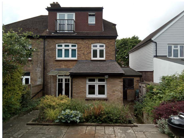
Figure 1: View from rear garden
