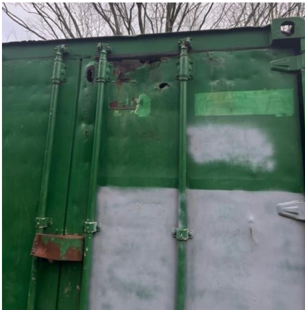
Image 1: Visible corrosion on the existing unit.
