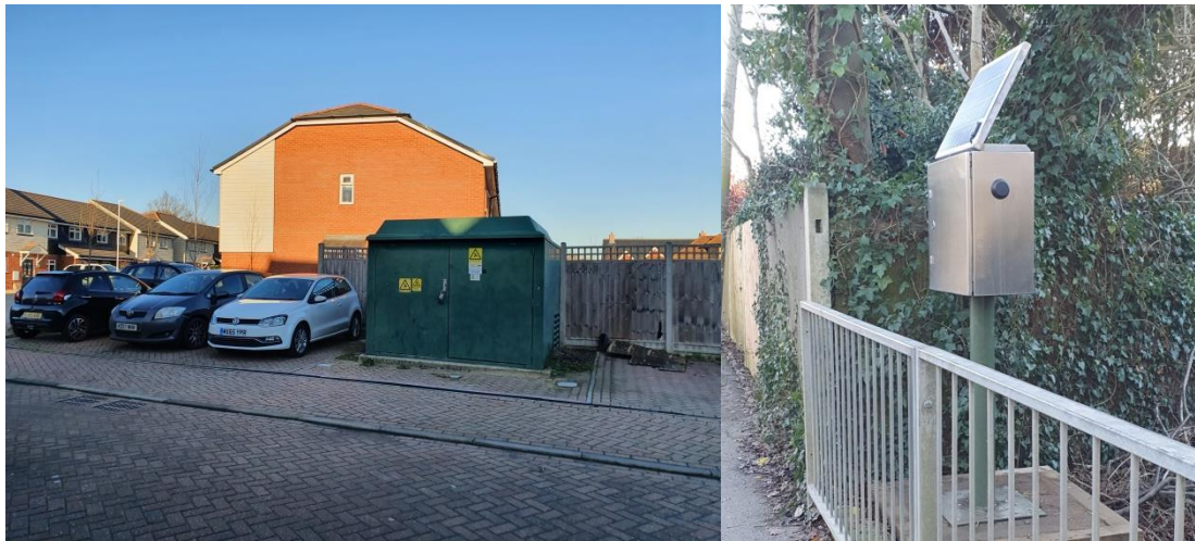
Figure 32: A bad and good example of integrating and visually screening utility infrastructure and equipment – the Hardwicks and Ulcombe Road
