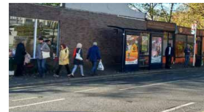
8.1 The west side of Sandling Road next to Maidstone East Station
