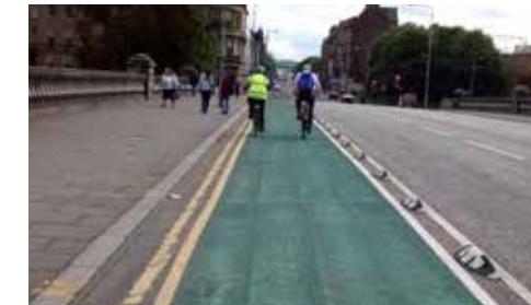
Example of light segregation Glasgow
