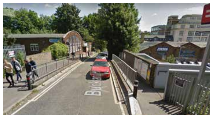
7.4 View east along Buckland Hill towards the river
