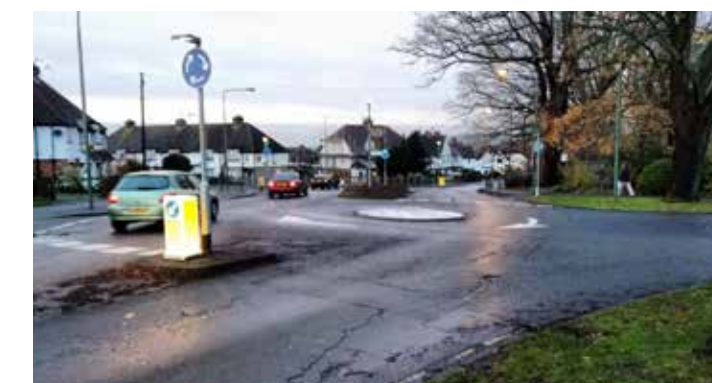
2.2 View north across double roundabout towards Willow Way
