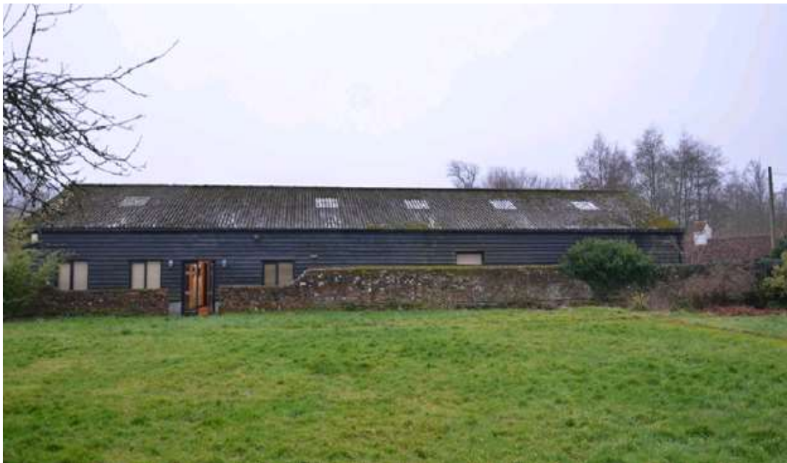
Figure 8 Rear elevation of the building viewed from the rear walled garden
