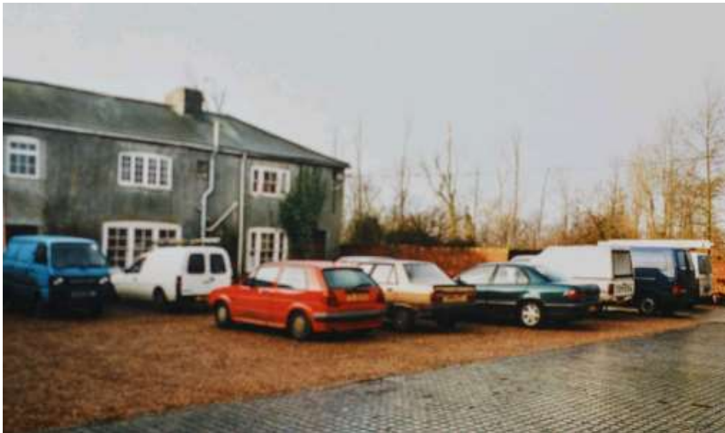
Figure 7: View looking west to Wells Cottage before and after improvement works
