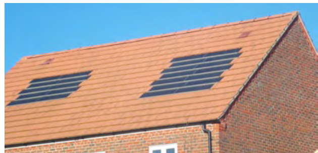
Recent development in North Loose with PV panels replacing tiles
