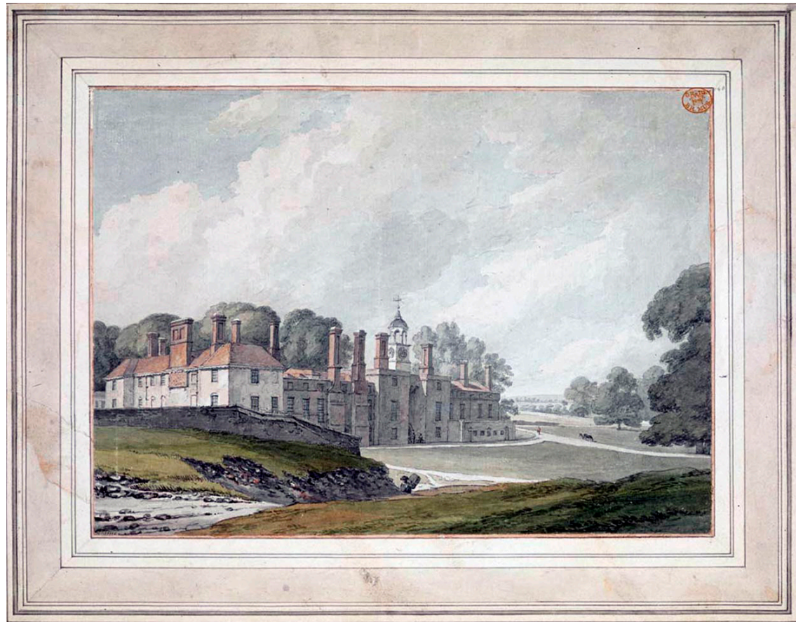
View of Mote Park shortly before demolition. Thomas Hearne F.S.A. (1744-1817)
