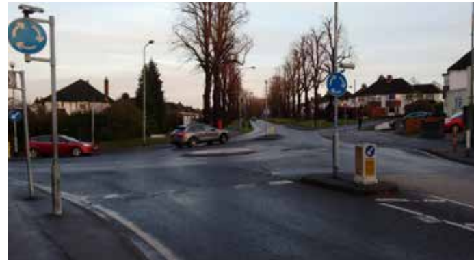
1.3 View of mini-roundabout looking west along Mote Road
