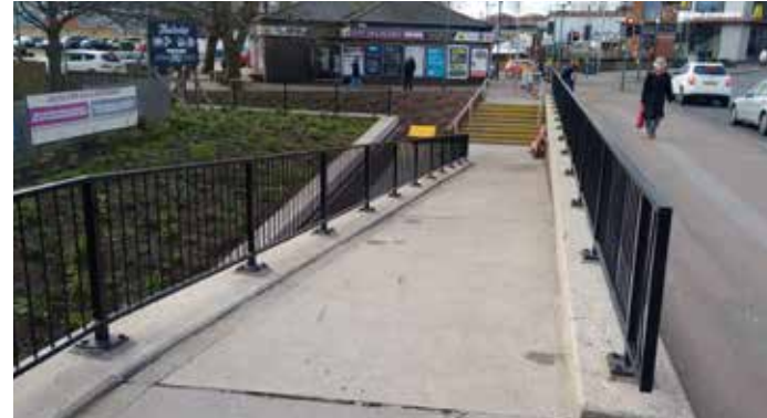
6.3 Access ramp to subway under the gyratory
