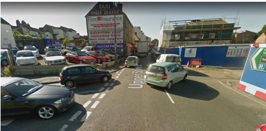
Figure 2-1: View of the north end of Upper Stone Street at the Wat Tyler Way/Knight rider Street junction (courtesy of Google Street View)
