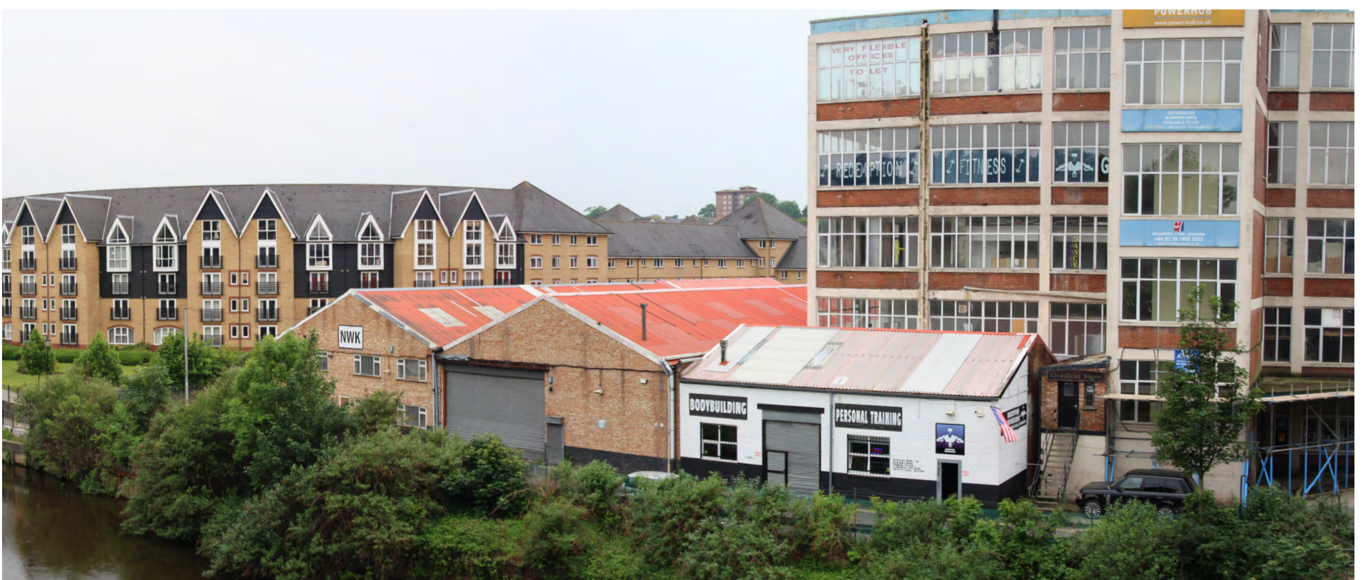
Powerhub site with Scotney Gardens beyond, seen from pedestrian footbridge over River Medway
