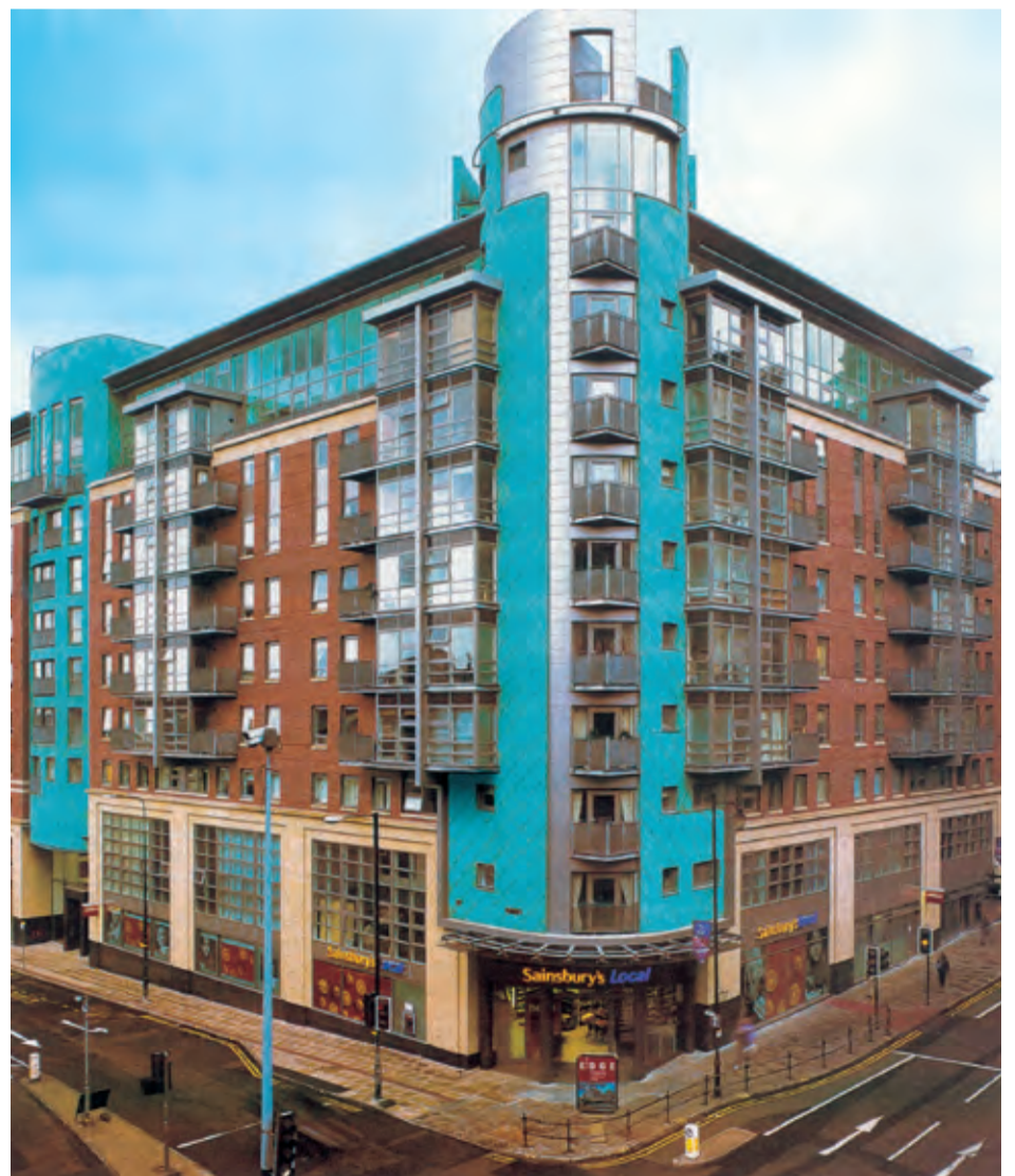
Apartments over supermarket within a landmark building
