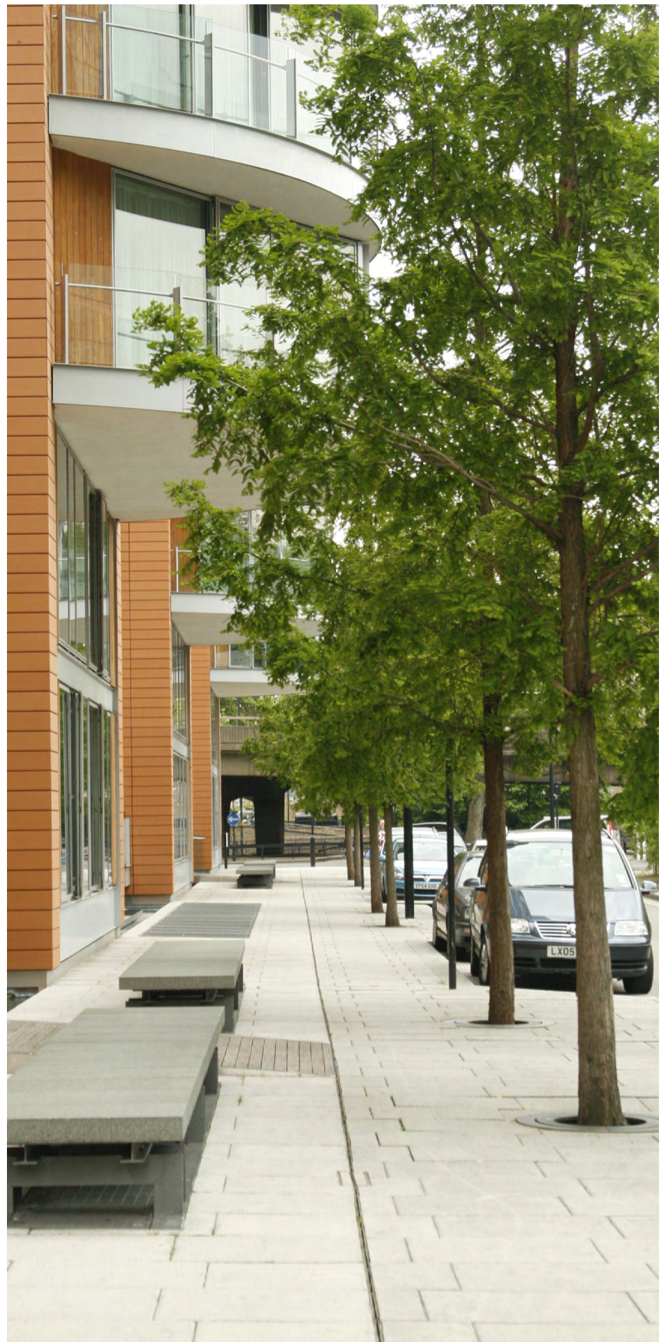
Building fenestration designed to allow informal surveillance of adjacent streets
