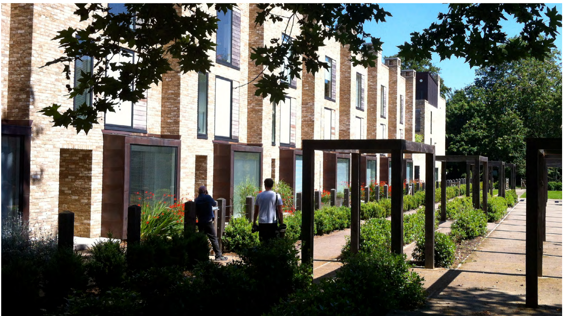
New development should be associated with low shrub planting to provide a green setting and privacy strip
