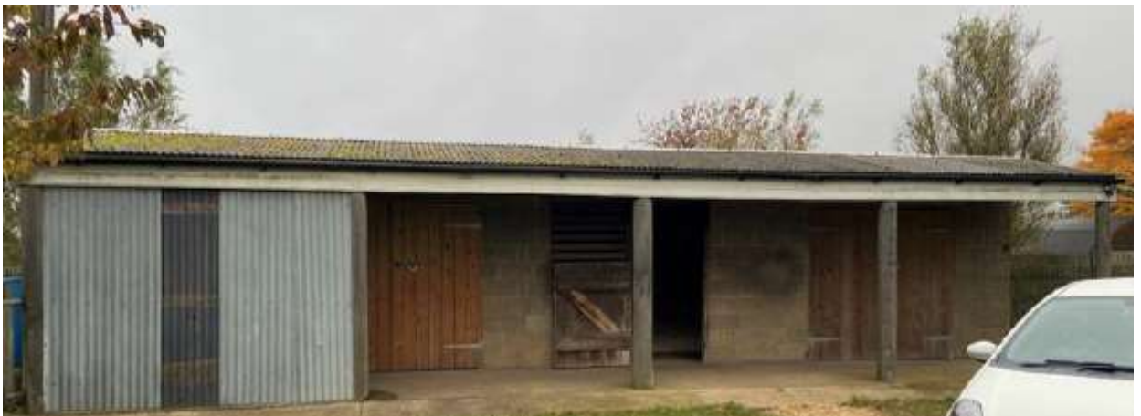
Existing Site Photograph
