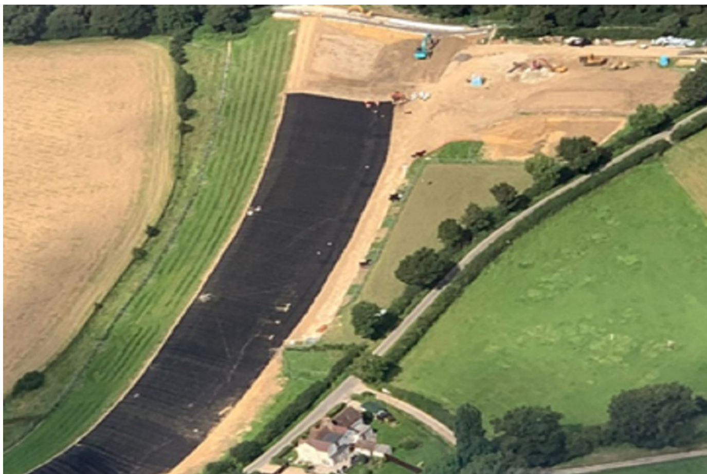
Laying the erosion matting at the first working area, summer 2021
