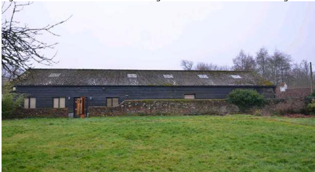
Figure 8 Rear elevation of the building viewed from the rear walled garden
