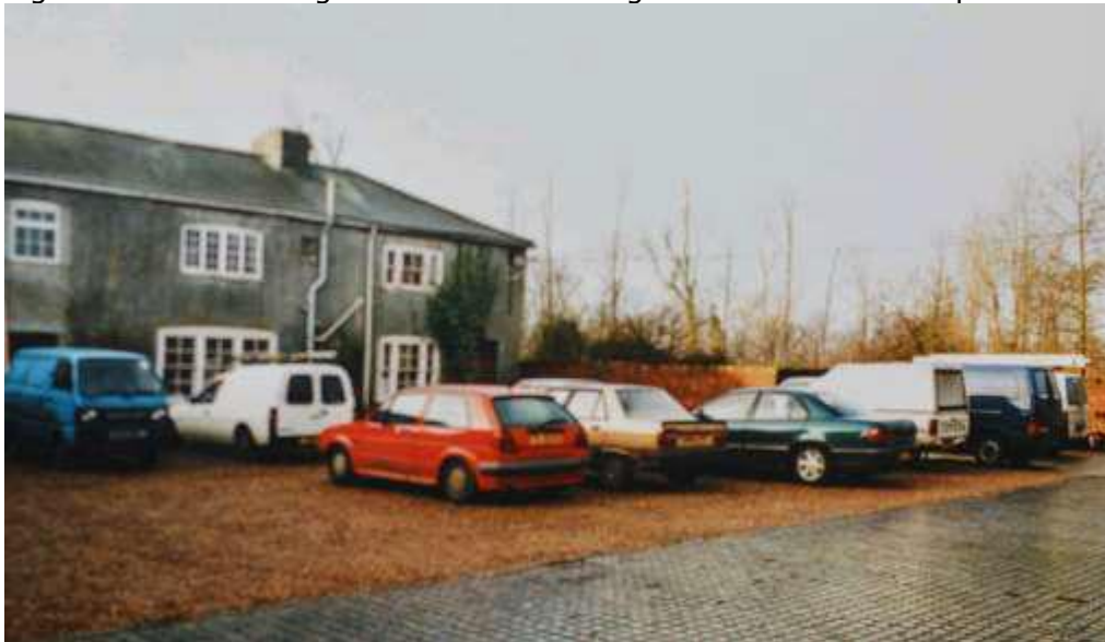
Figure 7: View looking west to Wells Cottage before and after improvement works
