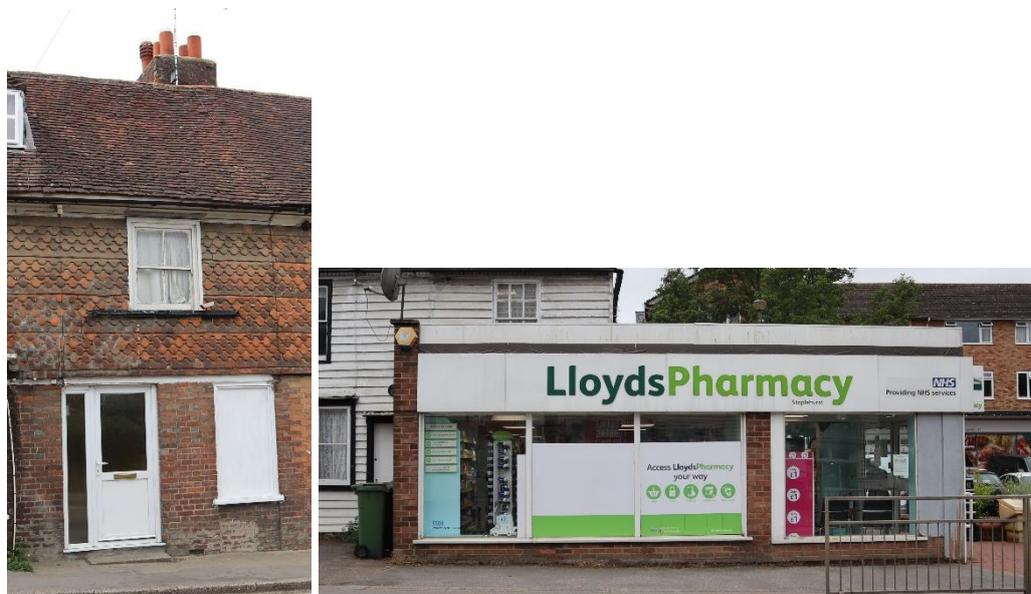
*Figure 48 – UPVc door (now replaced and blanked window to a traditional building and poor shop front which forms part of a listed building.*
