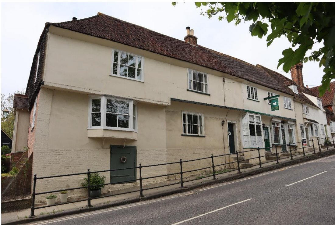
Figure 51 -painted render to timber framed properties.
