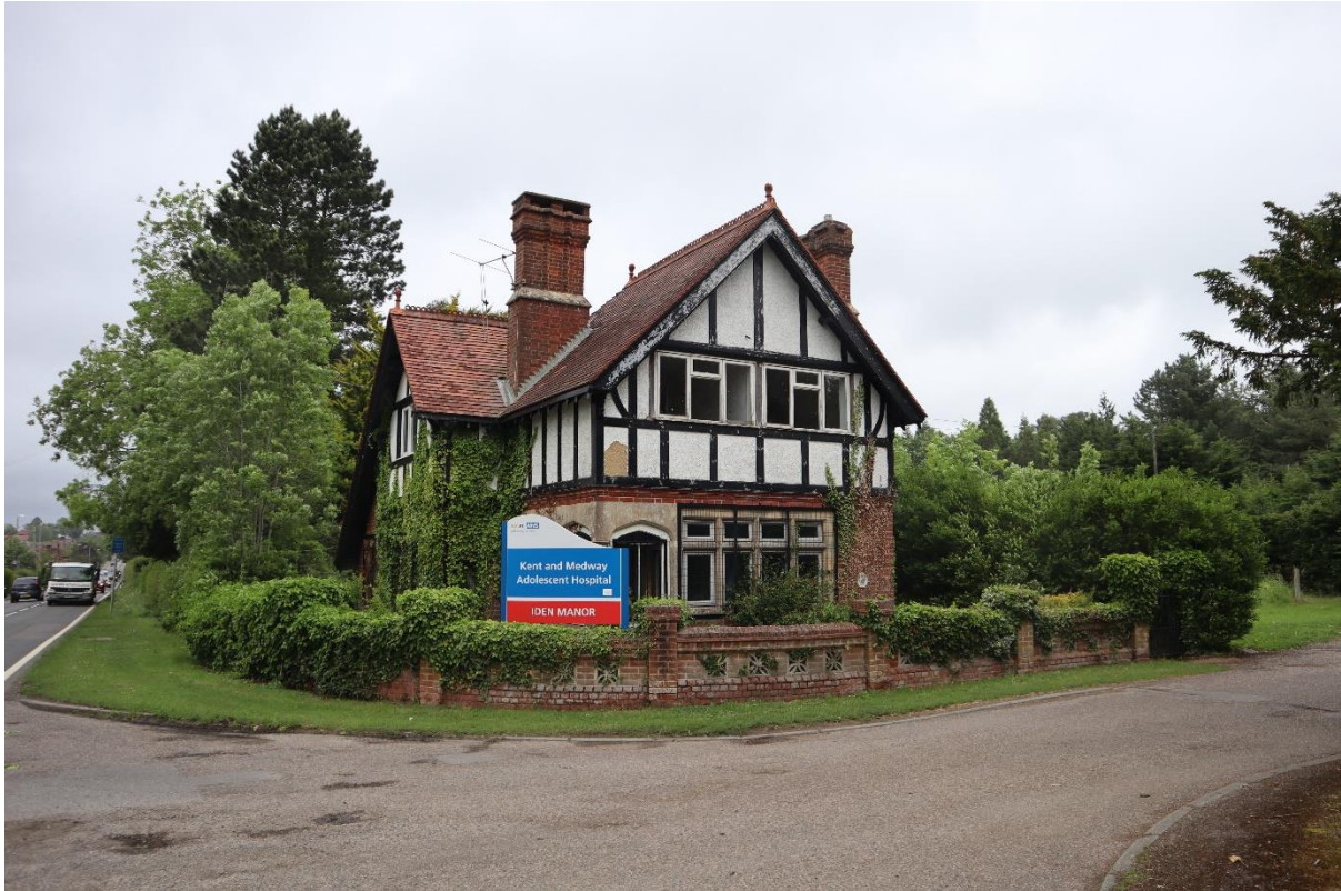
Figure 30 – Lodge to Iden Manor (at the time of the research was empty).
