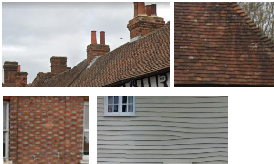
Figure 39 – examples of tiles, bricks, chimney stacks and weatherboarding.
