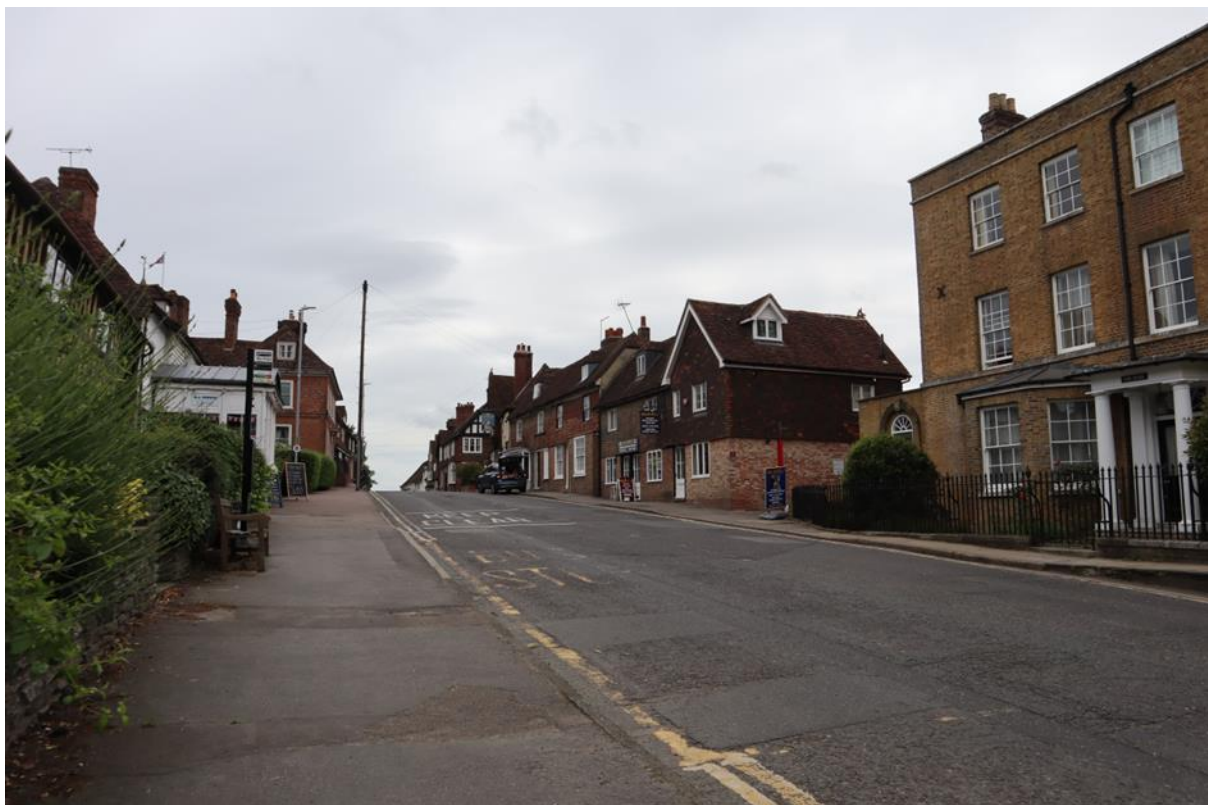
Figure 21 – The Limes, along High Street. The level of the road has been raised, street lighting removed and a change of the end of terrace. Bomb damage has resulted in some new development.
