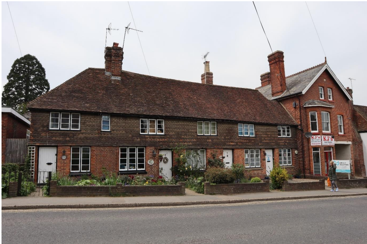
Figure 38 – Limes Terrace, with brick to the ground floor and hanging tiles to the first floor.
