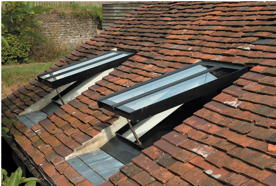
Figure 60 – example of a flush fitting rooflight – ‘Conservation Rooflight’.
