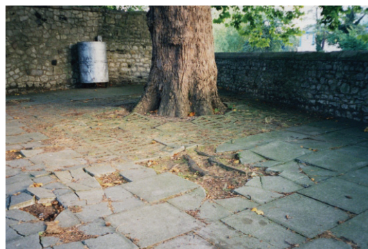
Surface roots can be a problem. Paving close to existing trees should be avoided as it presents maintenance problems and reduces important oxygen and water take-up.
