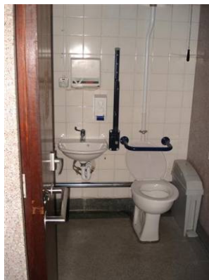
Church Street (bar on outside of door & high flush)
