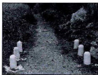
Back-up bollards make the barrier more visually imposing and less easily destroyed.
