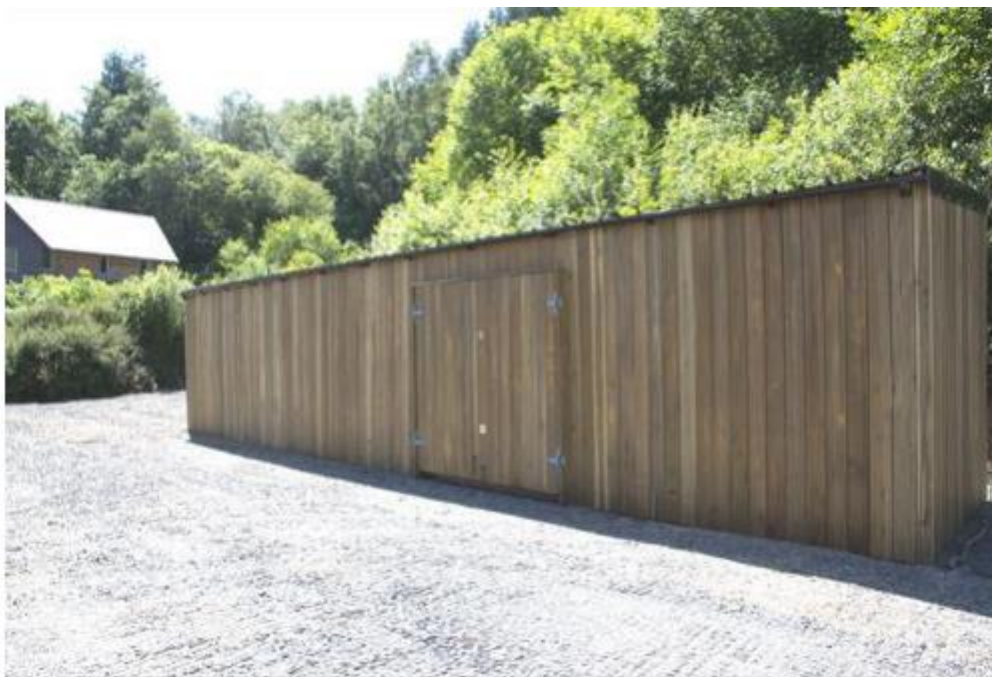
Figure. 1 Example of cladding
