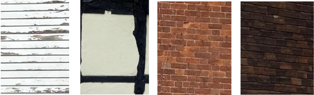
*Fig 20: Notable materials in the area include timber, weatherboard cladding, brickwork and tile hung cladding.*
