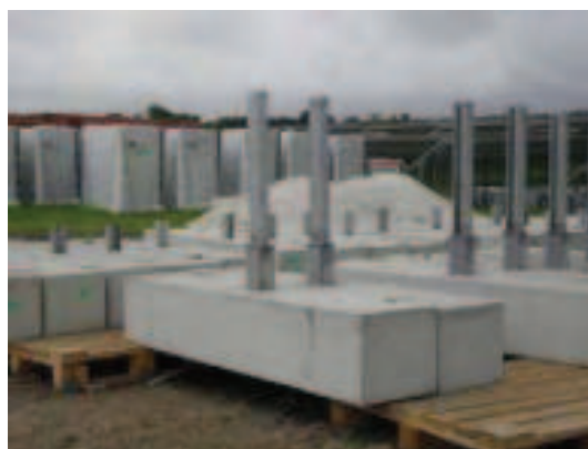
Where there are areas of archaeological interest and therefore a need to avoid ground disturbance, the use of pre-cast concrete anchors should be considered, as shown here at the 5MW Trefullock solar PV farm in Cornwall.
