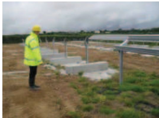
Where there are areas of archaeological interest and therefore a need to avoid ground disturbance, the use of pre-cast concrete anchors should be considered, as shown here at the 5MW Trefullock solar PV farm in Cornwall.
