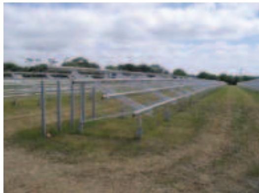
The ground anchors and framework associated with the development of the 1.4MW Benbole solar PV farm in Cornwall.
