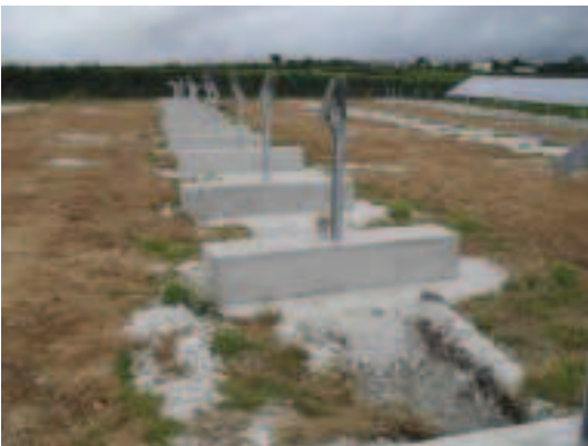
Where there are areas of archaeological interest and therefore a need to avoid ground disturbance, the use of pre-cast concrete anchors should be considered, as shown here at the 5MW Trefullock solar PV farm in Cornwall.
