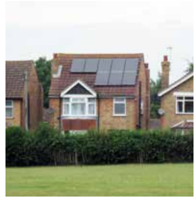
On-site energy generation is an issue that must be considered as part of the design quality assessment of any proposal.
