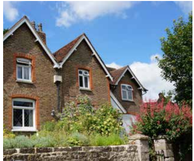
Protection of the built environment is a critical aspect of the plan (Objectives 1, 2, 5, 6 and 7).
