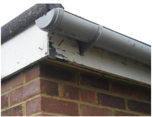
Photo no 5228 External Joinery to Club House - Weathered, use worn and defective
