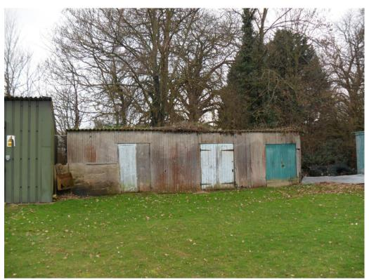
Photo 5200 Asbestos cement sports storage building- Dilapidated – To be removed
