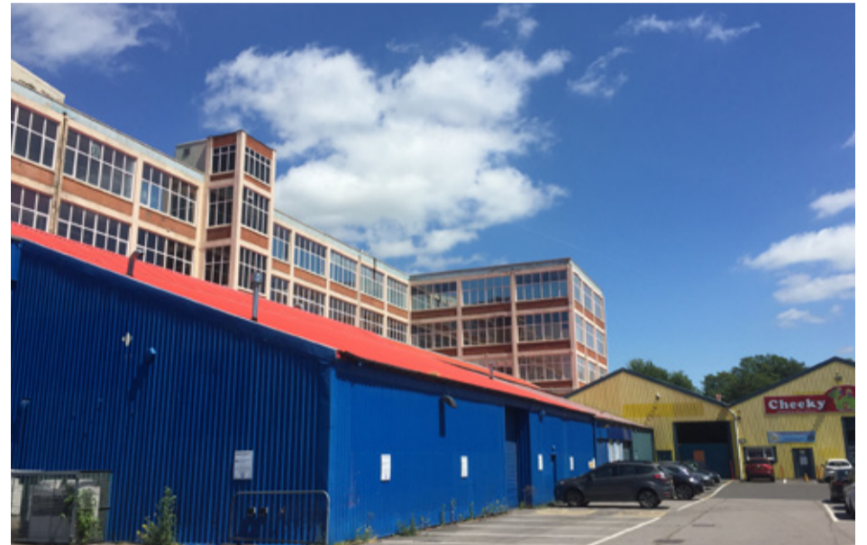
Powerhub/Baltic Wharf area: two to five storeys
