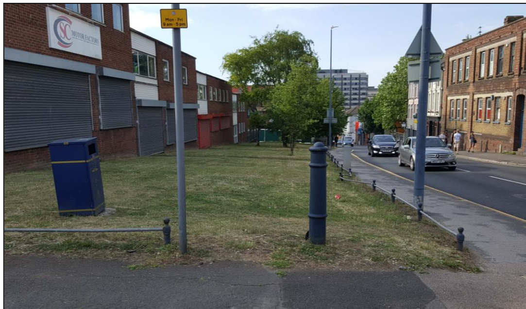
Figure 3.2 Existing GI Along Upper Stone Street
