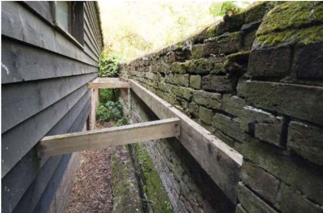
Figure 1 South wall curtilage lists showing existing propping
