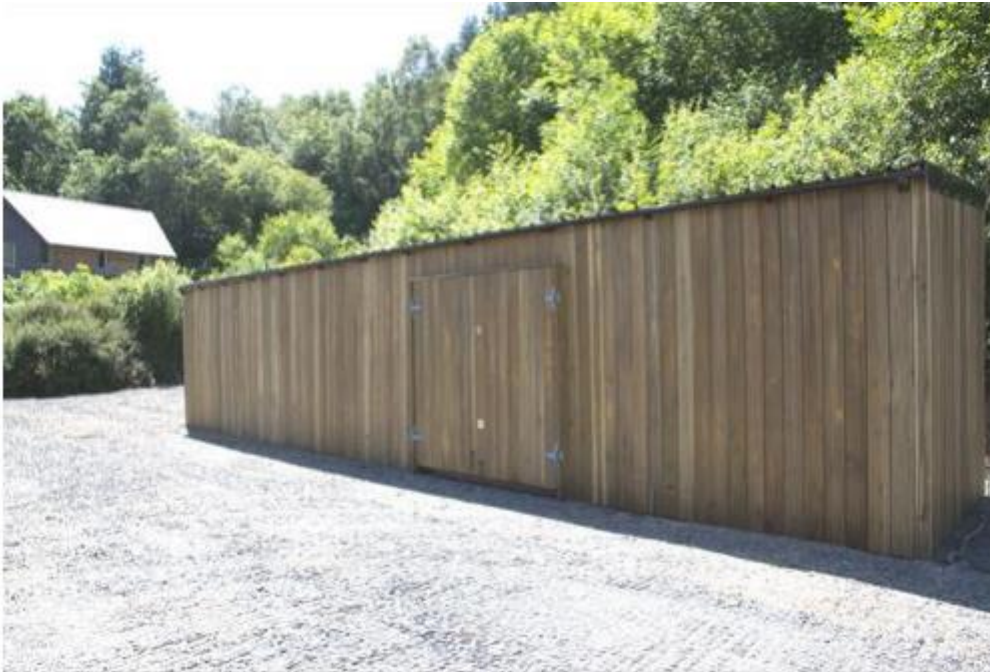
Figure. 1 Example of cladding
