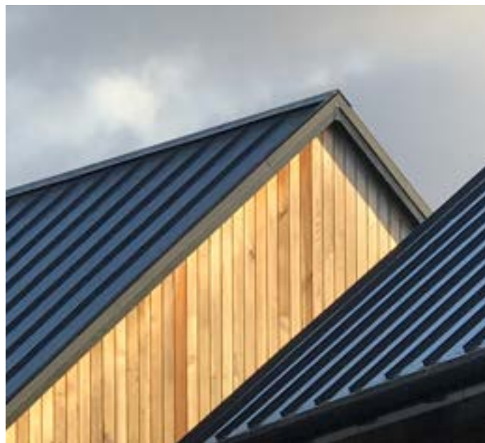
Pavilion Site- Standing Seam Roof
