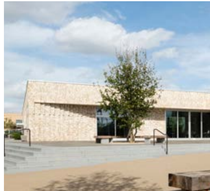
Heather House Site- Projecting Parapet
