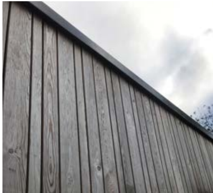
Heather House Site- Timber Cladding
