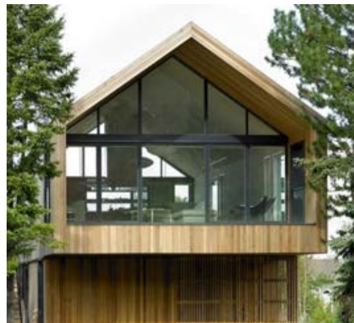
Pavilion Site- Gable Balcony
