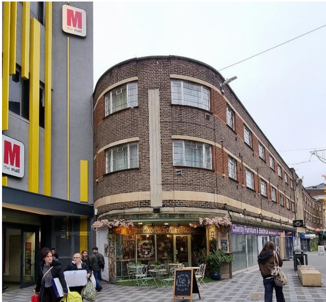
Figure 7 – Art Deco inspired building, with the Crittal windows above would suit metal shop front.
