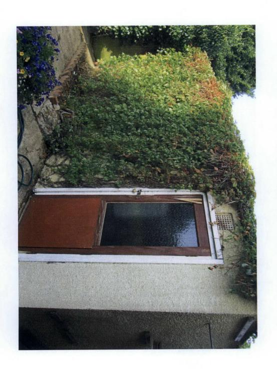
Size of out building 5.2M X 2.2M, Constructed using Breeze Blocks with rendered out side wall, flat roof construction.
