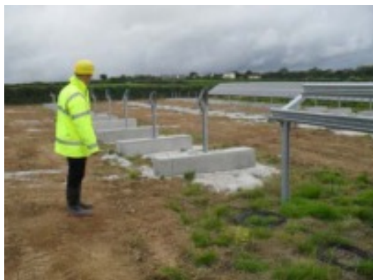
Where there are areas of archaeological interest, and therefore a need to avoid ground disturbance, the use of precast concrete anchors should be considered, as shown here at the 5MW Trefullock solar farm in Cornwall.
