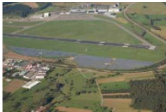
East Langford 5MW solar PV farm, Cornwall. Image courtesy of Low Carbon Solar.
