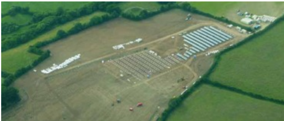
Construction of the 1.4MW solar PV farm on land adjacent to the Hendra Holiday Park, Newquay. Images courtesy of the Hendra Holiday Park.
