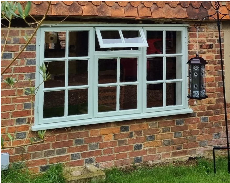
Figure 4 – whilst timber and single glazed, this is a modern storm window, with fanlight, within a listed building. These windows could be improved with flush casement windows without the fanlight.
