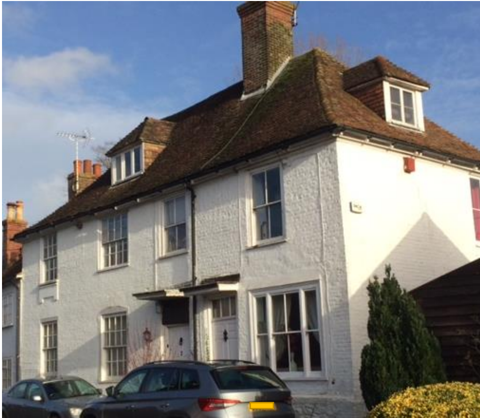
Figure 8 – different sash windows are shown here as the building has evolved.
