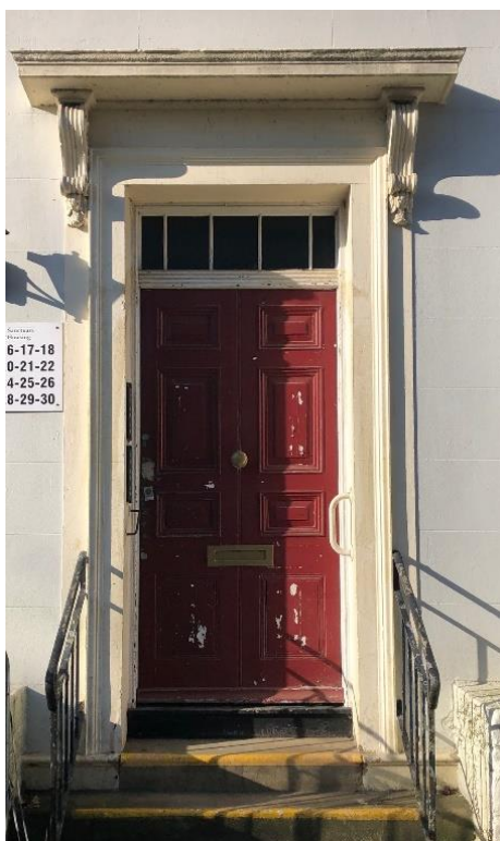
Figure 13 – an eight-panel door with a simple fanlight above.
