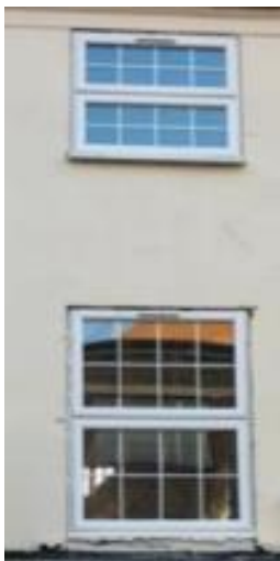
Figure 11 – large frames with inset glazing bars creates oblong details and flat finish.
