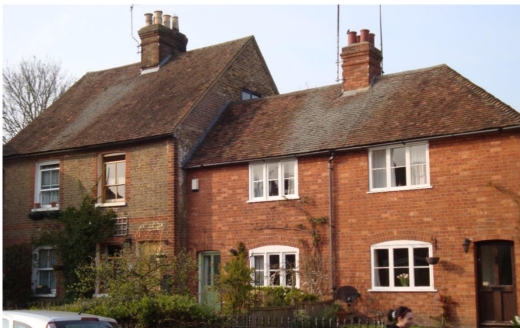
Figure 9 – sash windows to the cottage to the left, and casement windows to the cottage on the right.
