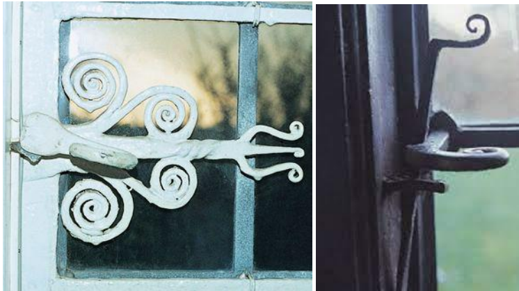
Figure 12 – early catches for casement windows.
