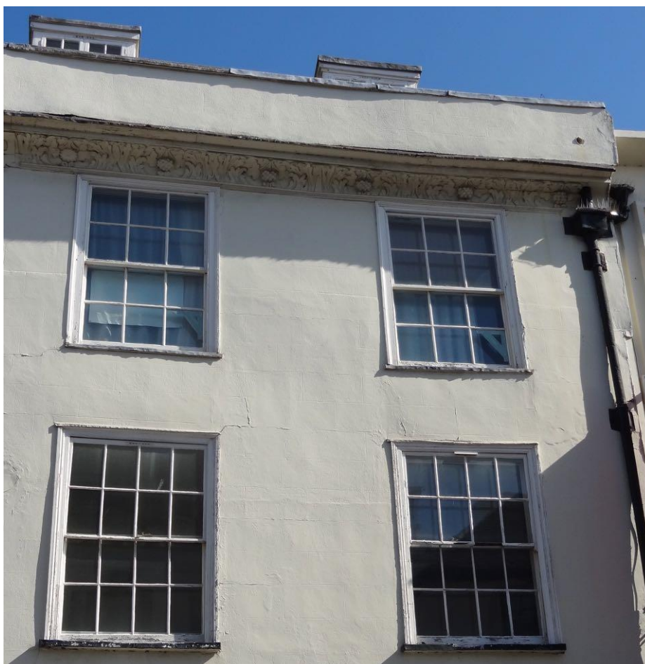
Figure 2 – original, single glazed sash windows, with casement windows to the dormers, contribute positively to the appearance of the property and the character of the conservation area.
