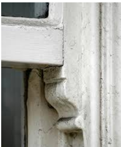
Figure 7 – horn to a sash window. These come in different styles.
