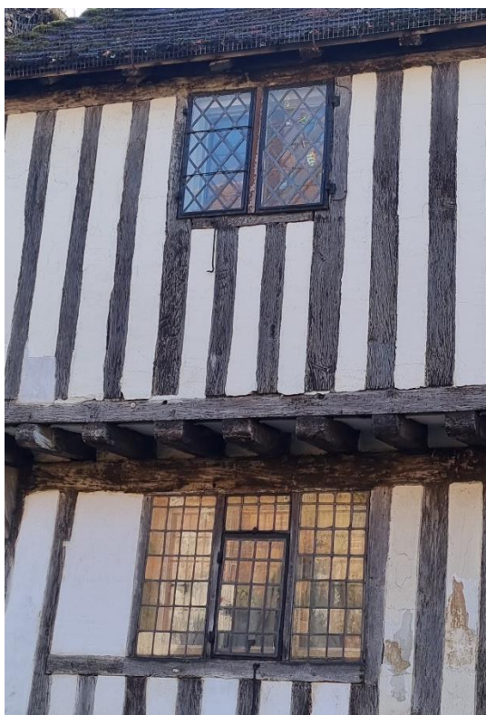
Figure 5 – metal framed, casement windows, with external hinges to the first floor and leaded windows. The ground floor window has been reduced in size.
