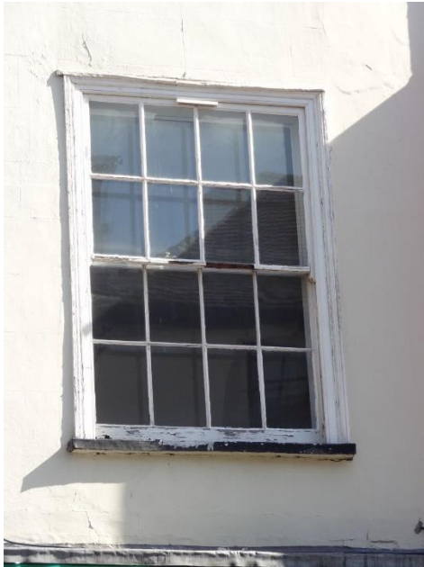
Figure 6 – whilst poorly maintained, this sash window has delicate glazing bars and mid-rails, showing that this is C18th.
