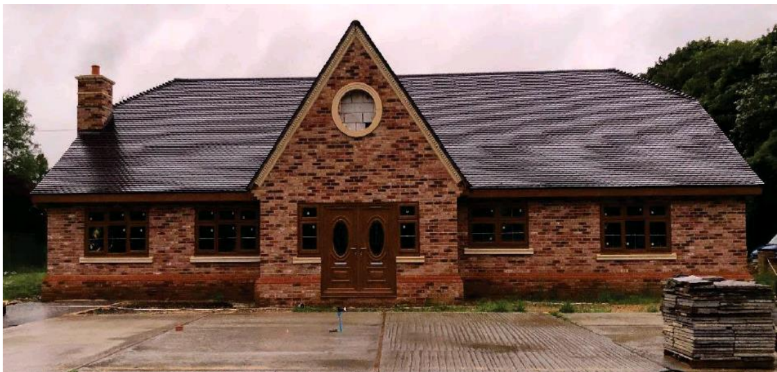
Figure 8: The front elevation of the existing building
